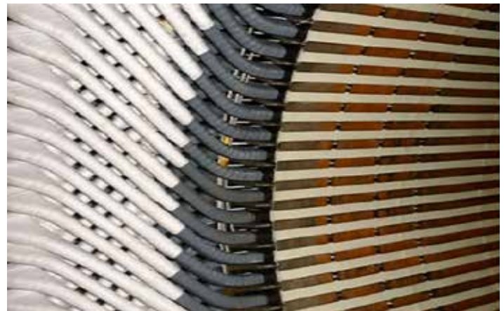
Figure 2. IE Medium and High Voltage Stator Winding
